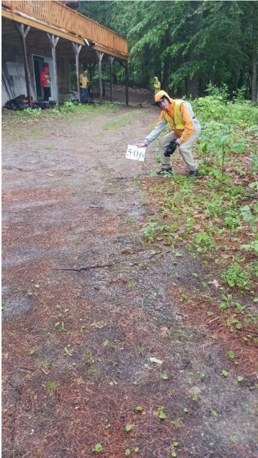
Figure 8: Example of surface erosion identified on a residential site.
