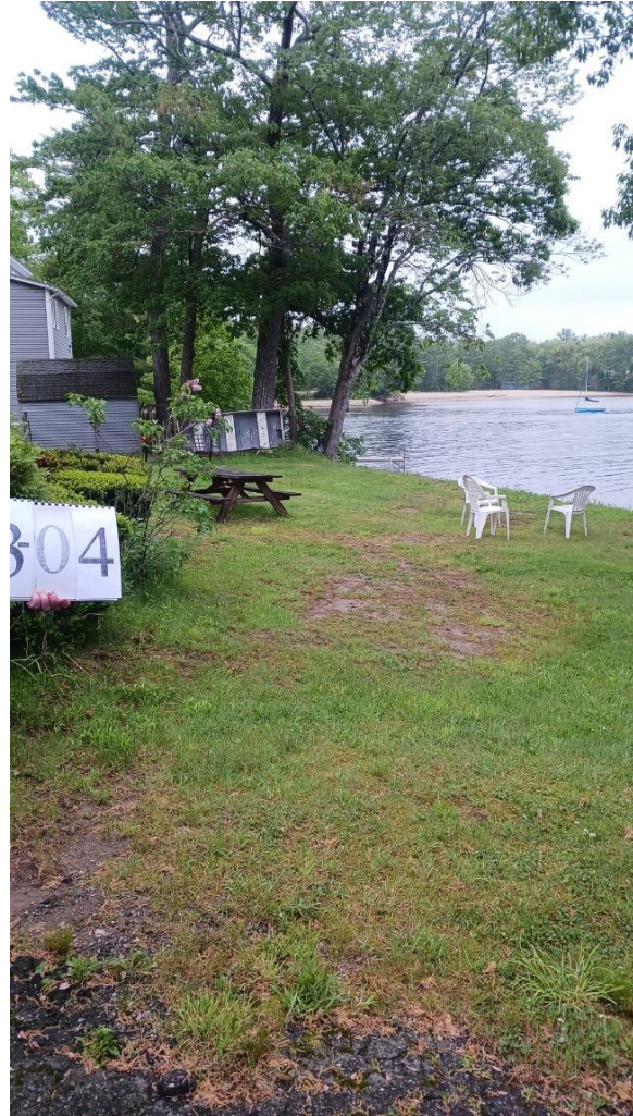
Figure 18: Low Impact Driveway Site Sheet Erosion leading directly to lake.
