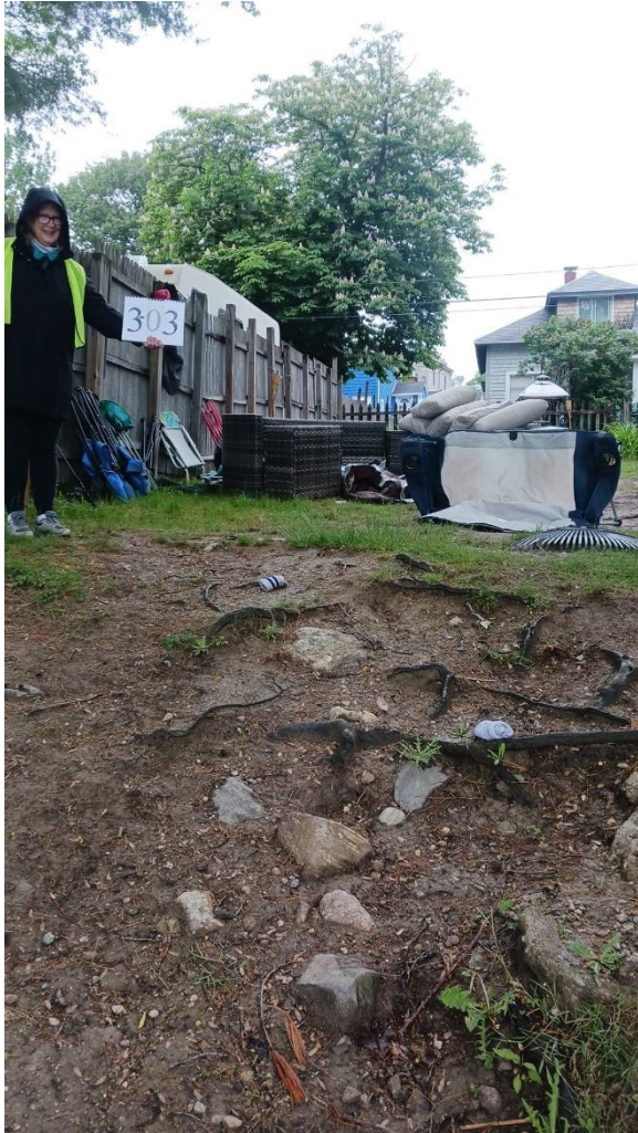
Figure 17: Low Impact Residential Site Sheet Erosion leading directly to lake.
