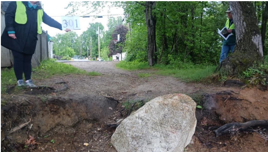
Figure 12: High-Impact Beach Access site
